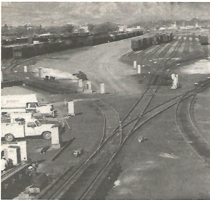
THE HUMP YARD at Grand Junction.
