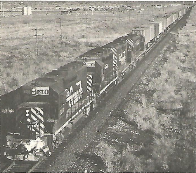
A RIO GRANDE TRAIN with loads of piggy backs highballs it to the west with four units on the head end, two GP 40s, a GP 35 and an SD 45, trailing 32 loads and three empties. Scene is near Grand Junction. (Cheedle photo)
