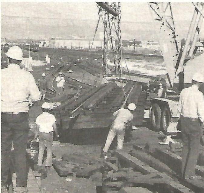
THE OLD RETARDER is lifted out of place.
