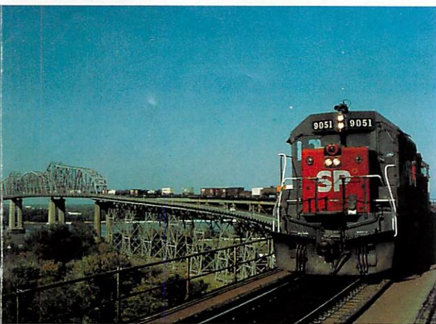
Huey P. Long Bridge at New Orleans. Photo by F. J. Famularo, cashier at Lafayette.
