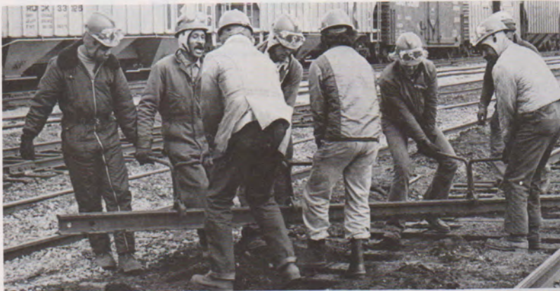
Tracks that the bankrupt Rock Island had been unable to maintain are rapidly being put back into service by the Cotton Belt. These MofW crewmen shown replacing a rail at Armourdale Yard in Kansas City are now Cotton Belt employees.
