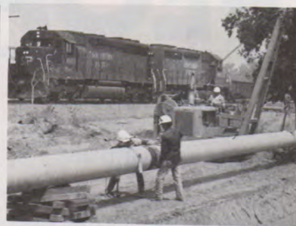
A new 20-inch pipeline was installed along SP railroad right-of-way.
