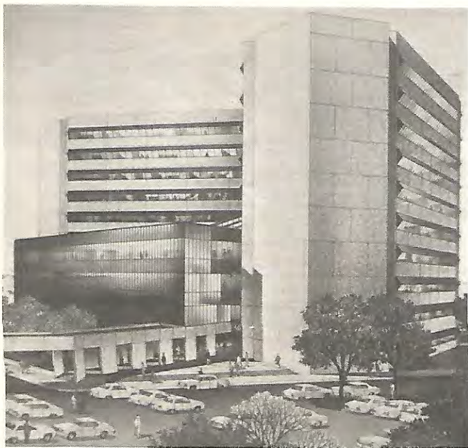
TEXACO, INC. will soon be moving into their headquarters at Bellaire, Texas. The 500,000 sq. ft. building will be composed of two 10-story towers adjoining each other at right angles. In designing the building, consideration was given to reducing the amount of energy necessary to operate it. Insulated walls, shaded windows and reflecting glass will reduce the heating and air-conditioning load. The new building will enable Texaco to consolidate virtually all of its operations and provide future expansion space as needed.
