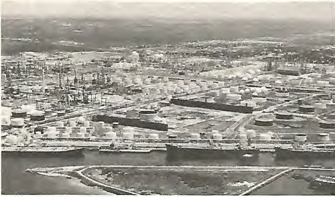
SHELL OIL COMPANY, Houston, Texas has eight refineries in the United States. Their total capacity is about 1,085,000 barrels per day, making hundreds of petroleum products from gasoline to jet fuel to wax and asphalt. Their chemical plants manufacture the basic petrochemicals which are processed by others into plastics, resin and pharmaceutical consumer products. Shell Manufacturing Plant, Deer Park, Texas, in the photo, as seen from the loading dock facilities on the Houston Ship Channel where tankers from over the world bring crude oil to be processed.
