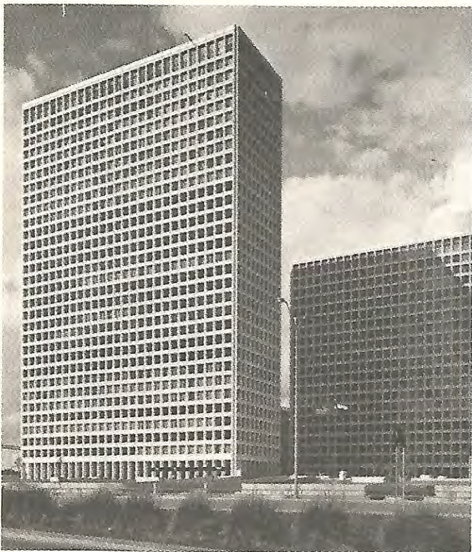
CONTINENTAL OIL CO., with Western Hemisphere Petroleum Division headquarters at Houston, Texas, is a world-wide company having varied interests in petroleum, pipeline, coal, chemicals and plastics and other energy related endeavors. This firm plays a vital role in the research, exploration, development and marketing of energy needs for our nation and employs nearly 40,000 persons. Conoco celebrated its 100th anniversary in 1975.
