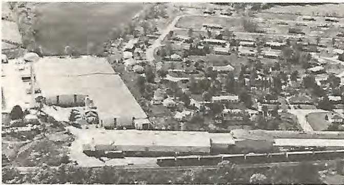
PERMANEER CORPORATION, St. Louis based manufacturer, converts wood chips and vinyl film into attractive building materials and furniture products. Over the past five years, the company has become one of the most important factors in its industry. Utilizing a low cost wood substrate, Permaneer is able to serve segments of established multi-hundred million dollar markets which cannot be economically supplied by traditional manufacturing techniques. Permaneer's unique technical manufacturing abilities provides the answer to the high cost and shortage of natural hardwood and skilled labor. (Wright City, Mo. plant shown)
