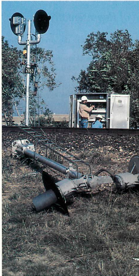
New CTC signals have three separate lenses mounted within the circular black area and replace the old style (foreground) which used only one lens.
