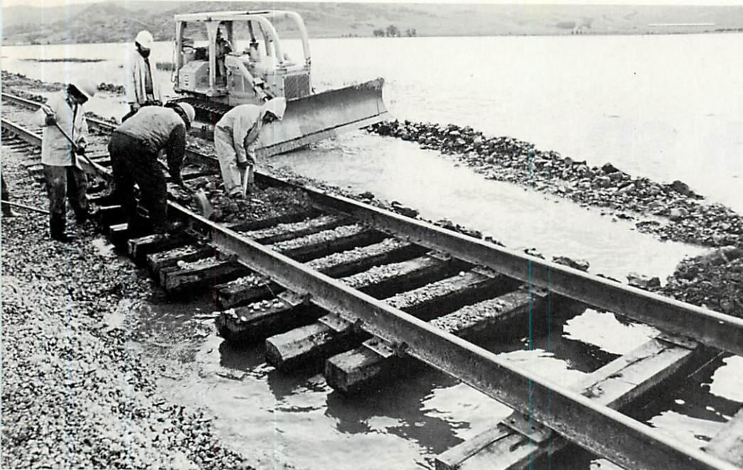
At Bahia, between Oakland and Sacramento, workers prepare to add riprap and ballast to track damaged by high winds and water in the Sacramento Delta.
