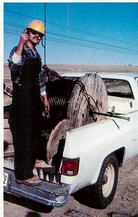
Signalman Rodney Leard works on the siding extension at Vaughn.
